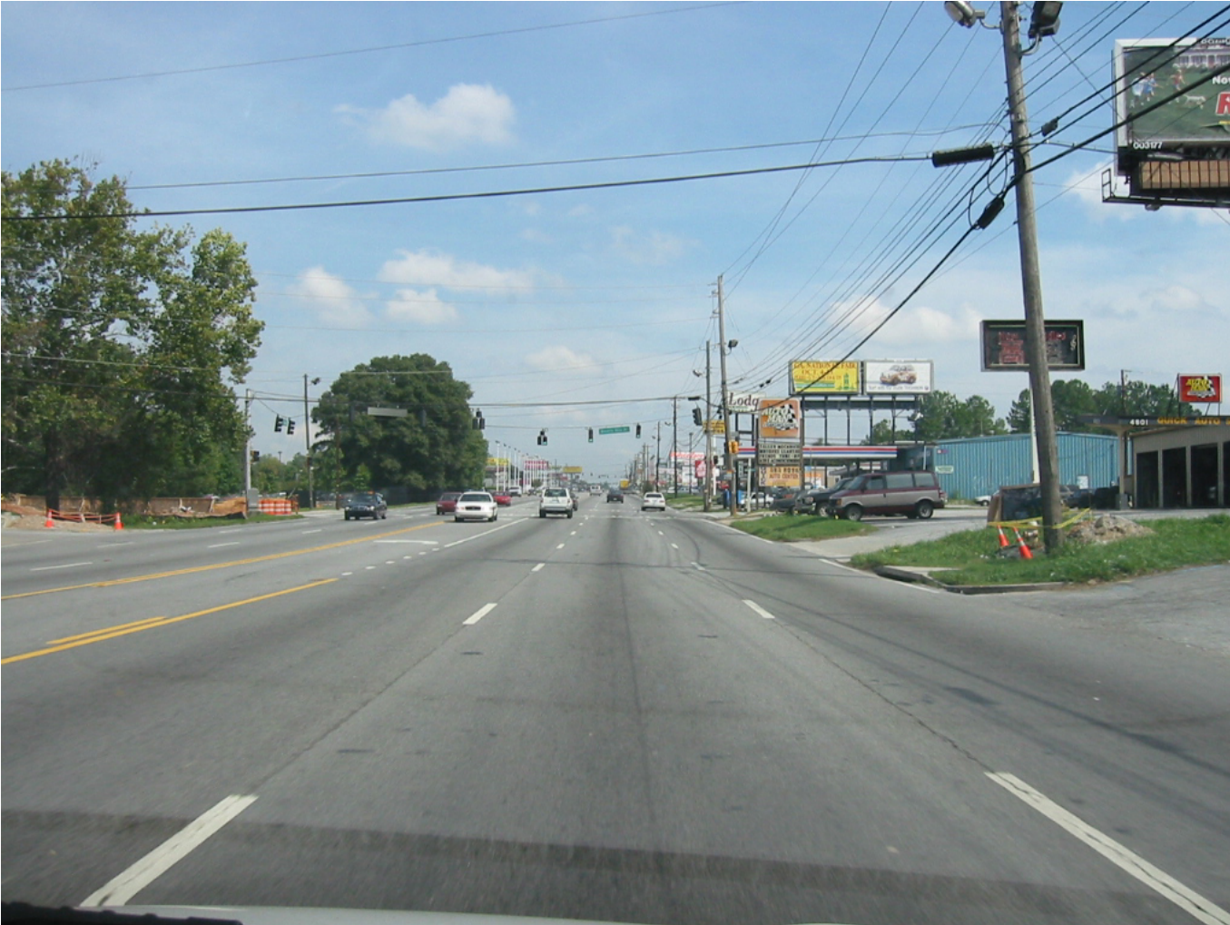
Photo courtesy Michael Gamble, Georgia Tech School of Architecture
